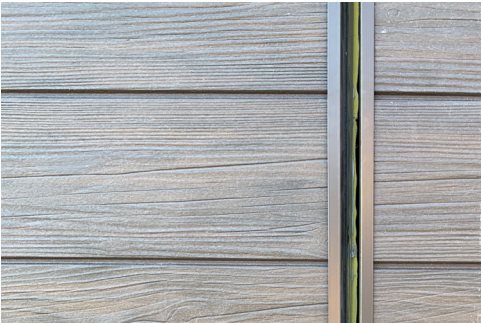
Vertical Unit Joint at jobsite prior to the addition of sealant.
